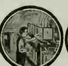
STORAGE BATTERY SYSTEM
