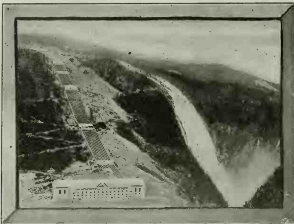
The Above View Shows the Gigantic Hydro-Electric Generating Station for the Fixation of Atmospheric Nitrogen at Rjukan, Norway. The Great Power of this Station can be Appreciated by Noting the Large Number of High-Pressure Water Pipes Leading Down to the Electric Generating Station, and Which By-Pass the Necessary Water From the Large Waterfall. The Station Is the Largest in the World and Develops 250,000 Horse-Power.
