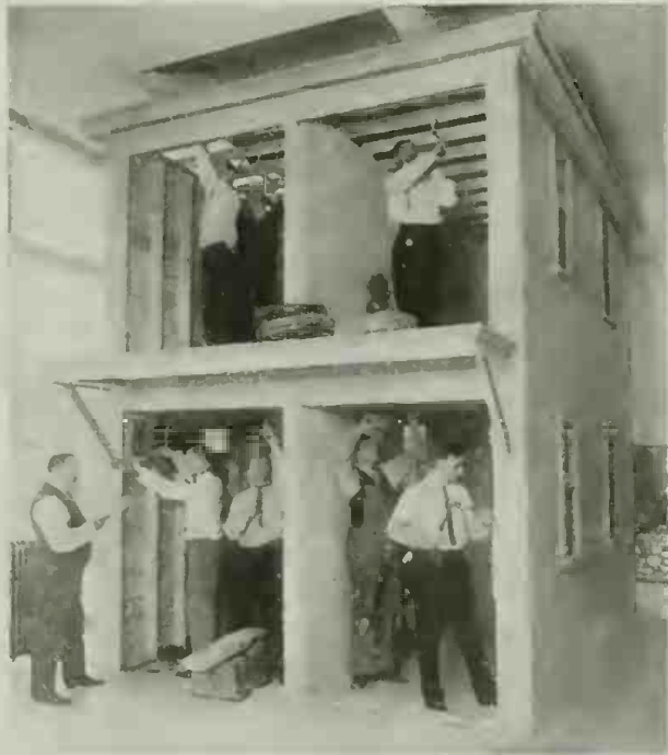
Students Completely Wiring Model House in School
